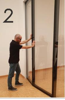
Push the frame as seen in the image on the left until the panels are parallel with the rail.
